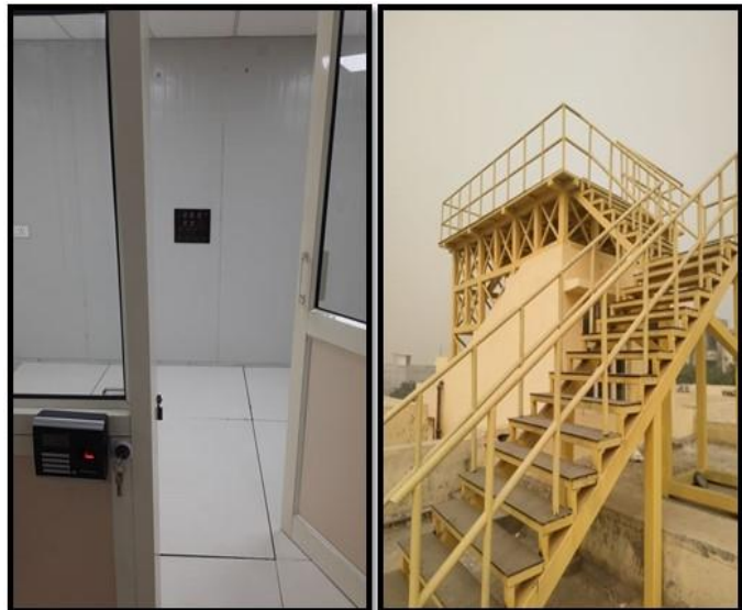
Newly established Time laboratory at RRSL Faridabad and antenna structure for mounting GNSS antennae for the time link
